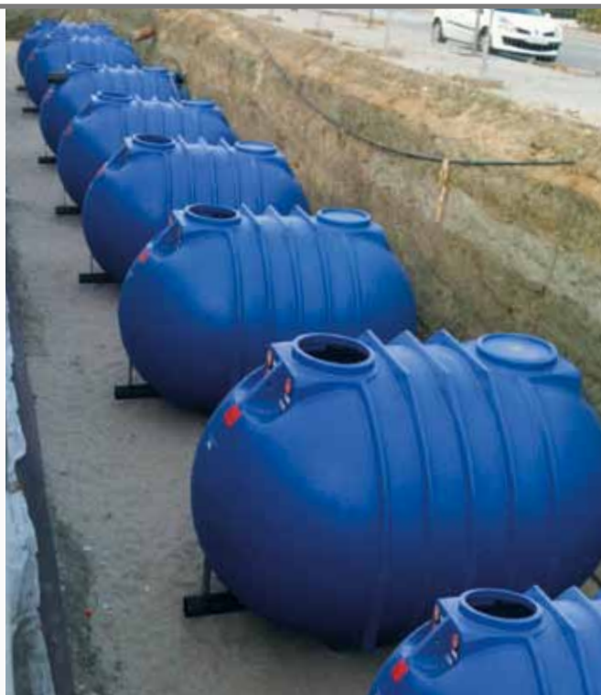
Installation with Underground BlueLine II Tanks : Example : BlueLine II 80000 litre Installation (8 x BLII 10000 litre)
